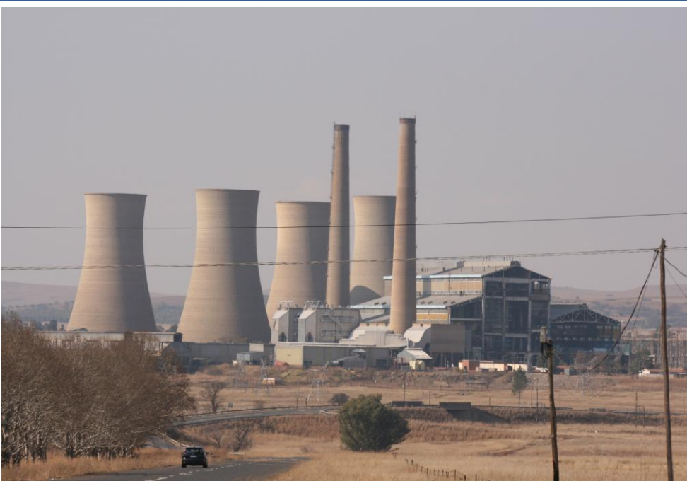
Photo 2: Power Station just outside Newcastle
